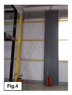
**4** Use bagged ropes to keep the worksite tidy and ensure there is enough rope in the bags to lower the casualty to the ground. **Fig.5**  Equipment for Rope Access
