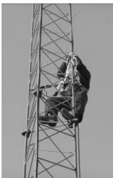
Primary support: Tower structure Fall protection: Fall arrest lanyards ('twin tailed')
