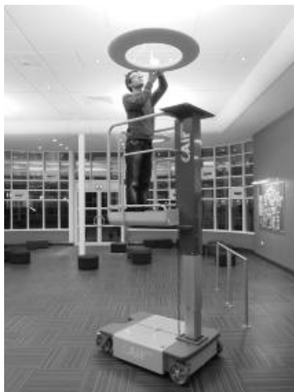
Primary support: MEWP Fall protection: Platform guardrail
