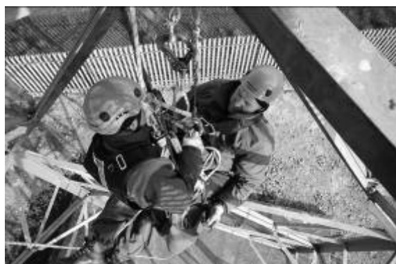
Primary support: Casualty's deployed lanyard Fall protection: None
