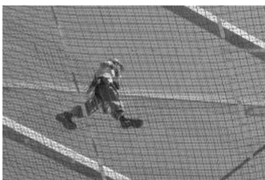
Primary support: Walk-on netting Fall protection: Secondary safety netting (below)
