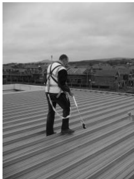
Primary support: Rooftop Fall protection: Permanent horizontal anchor line (fall arrest system)
