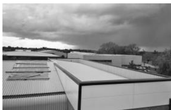
Primary support: Roof top Fall protection: Raised edge
