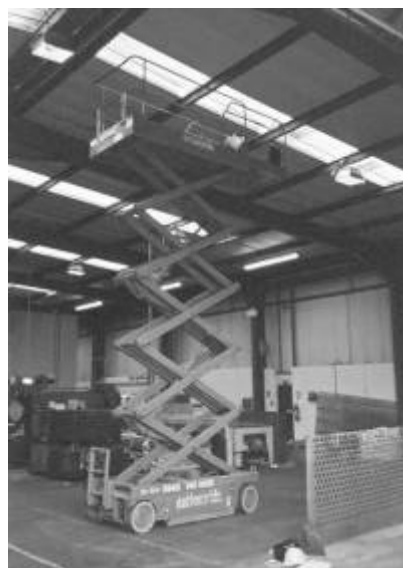
Primary support: MEWP (Scissor lift) Fall protection: MEWP basket
