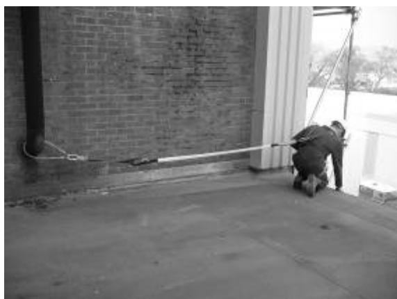
Primary support: Rooftop Fall protection: Restraint lanyard
