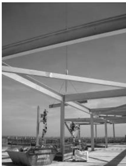
Primary support: MEWPs from floor slab Fall protection: MEWP basket (and restraint lanyard)
