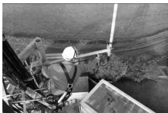
Primary support: Work restraint lanyard (and legs) Fall protection: Fall arrest lanyard
