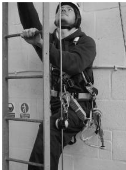
Primary support: Ladder stiles Fall protection: Vertical fall arrest system ('slider')
