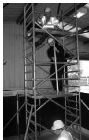
Primary support: Platform Fall protection: Guardrails
