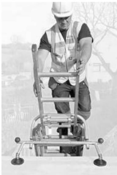
Use of a ladder (with a stability device) – 'bottom of the hierarchy'
