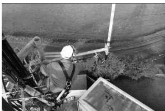
Minimising distance and consequences (work positioning with fall arrest back-up) – Individual protection
